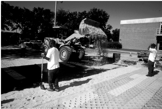
Figure 2. Parking lot under construction. In foreground, a Turfstone™ concrete block paver layer is laid. Underneath in succeeding order is bedding sand, a permeable fabric and a marl subbase.
