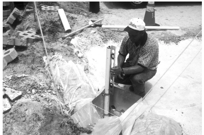
Figure 6. Installation of flume stick in weir box. The height of water over the nape of the weir is used to determine volume of runoff from the parking lot.
