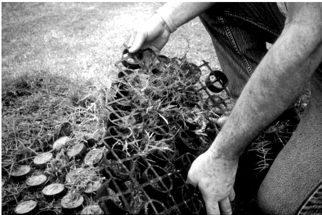
Figure 4. Bermuda grass roots visible in plastic grid paver.
