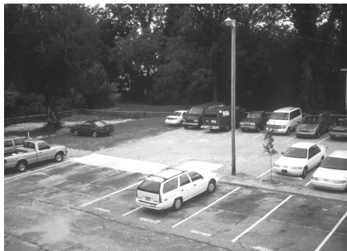
Figure 1. Permeable pavement lot at Alice Hannibal Building in Kinston, NC. Far left-hand side of lot is re-inforced grass. Far right-hand side is concrete modular block filled with sand. Lot in foreground is asphalt.
