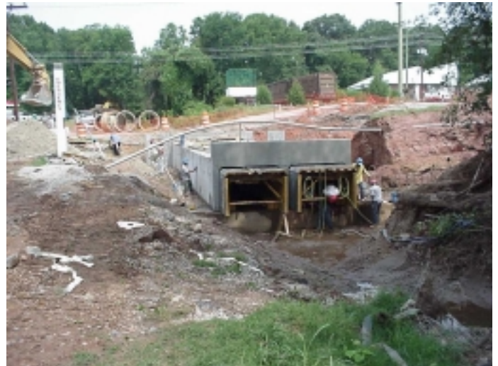
Figure 7. Culvert replacement at Rocky Branch.
