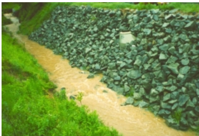
Figure 6. Riprap placed in Rocky Branch during previous attempts to stabilize the banks. This is another example of traditional stream armoring.
