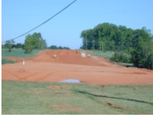
Figure 5: Construction of I-485 Bypass in Goose Creek watershed
