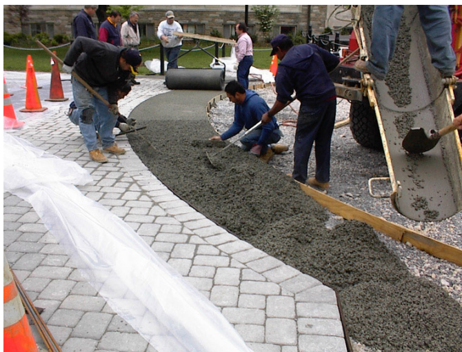
Figure 7: Pouring of porous concrete. Drum roller used for compaction and finishing.
