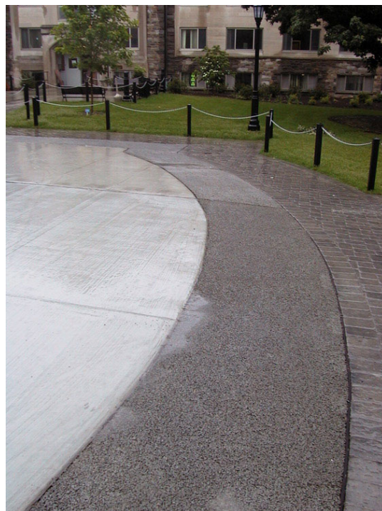
Figure 6: Runoff being infiltrated by porous concrete.
