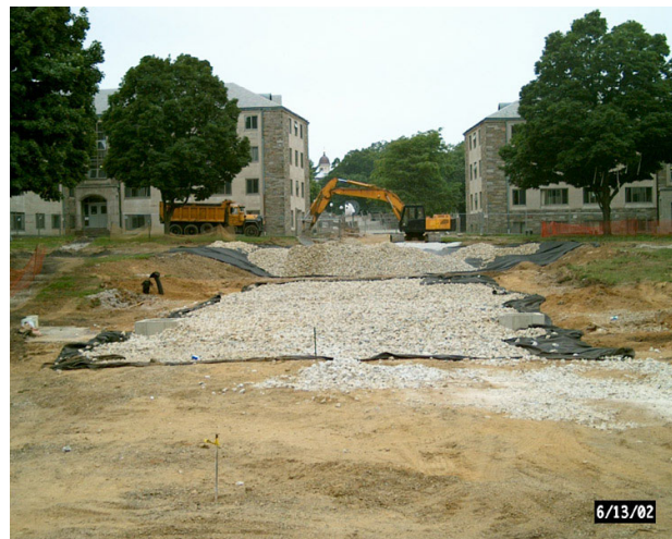
Figure 5: Construction of porous concrete infiltration beds with #4 baffle stone in place.
