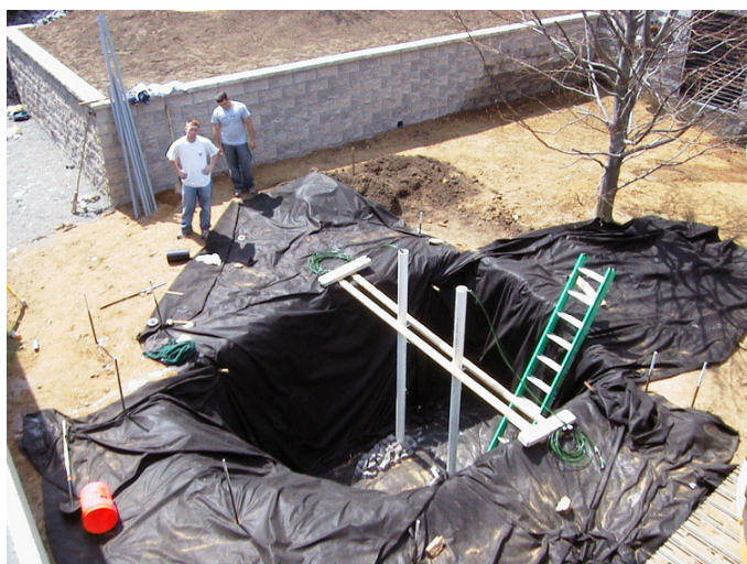
Figure 8: Completion of trench excavation with geotextile fabric lining. Note locations of the two monitoring wells.
