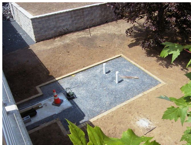
Figure 9: Completion of trench prior to application of eco-pavers. Trench was filled with washed crushed stone, and perforated distribution pipe was installed.
