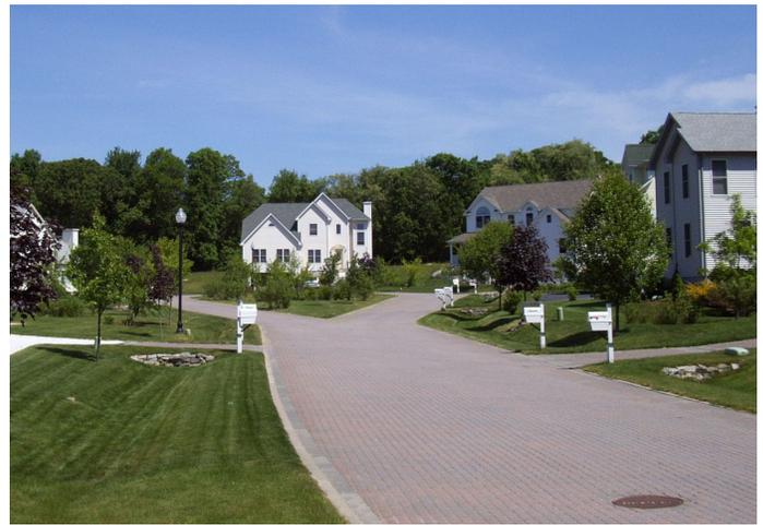
**Figure 4.** Photograph of BMP portion of the Jordan Cove Urban Watershed NMP Project showing a grassed swale, concrete paver road, and the bioretention cul-de-sac.
