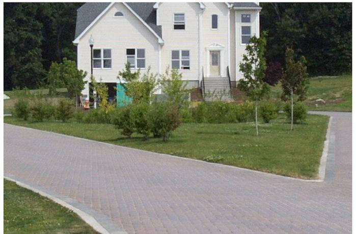
**Figure 5.** Photograph of the bioretention cul-de-sac at the Jordan Cove NMP project.
