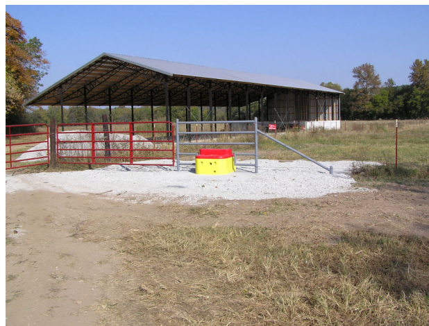
Figure 7. Winter feeding facilities with waste storage capabilities were effective at reducing the amount of soil erosion and nutrient runoff.
