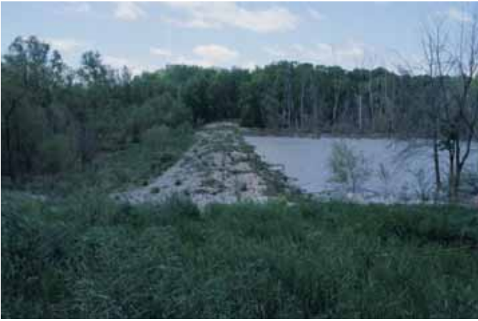
Figure 5. A large sediment retention basin (SRB) constructed just upstream of monitoring station B and Lake Pittsfield served as a final sediment treatment with an estimated 80 to 91% sediment trapping efficiency. Today, the SRB also provides valuable wetland habitat.
