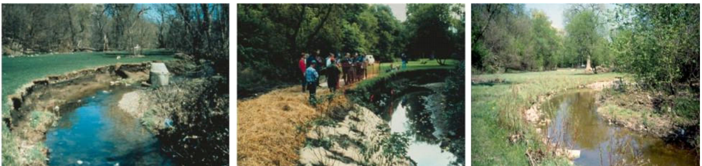
Figure 11. Stream restoration at station S1 show pre-restoration conditions before 1991 (photo on left), mid-restoration condition in 1994 (middle photo) and post-restoration conditions in 1995 (photo on right).
