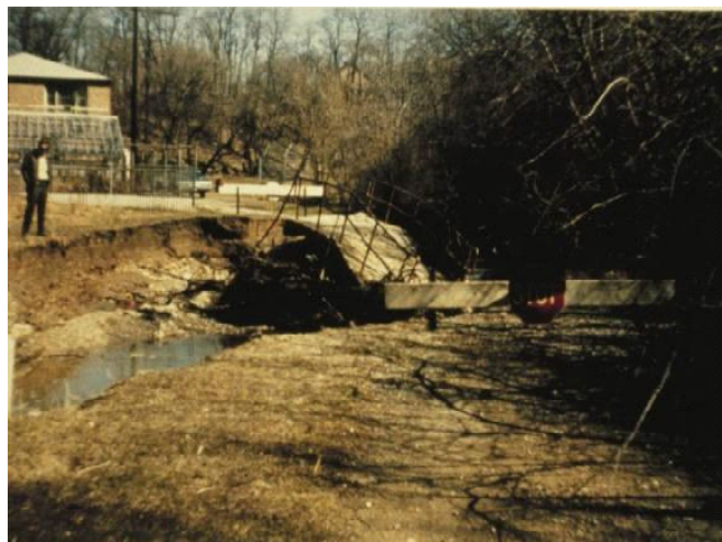
Figure 4. Damaged infrastructure on the South Branch from “flashy” storm events in 1990 in Washington Park.
