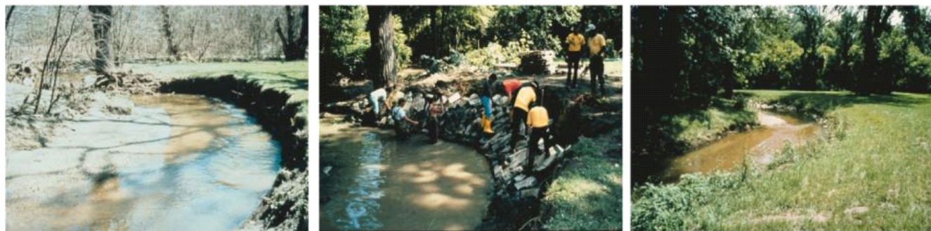
Figure 9. Stream restoration applied at station N1 before restoration in 1991 (photo on left), during construction in 1992 (middle photo), and post-restoration in 1993 (photo on right).
