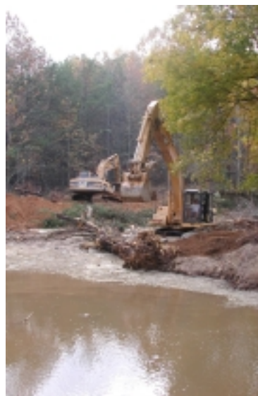
Fig 5: Building a pond in Reach 4
