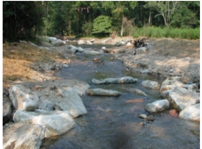
Fig 4: Looking upstream in Reach 2, two log and rock cross vanes in the new channel
