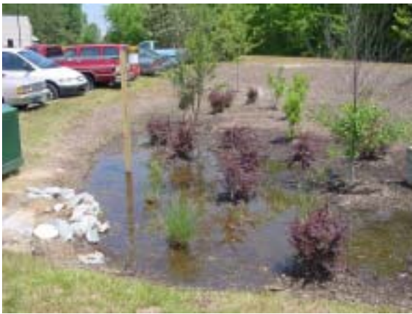
Figure 7. Bio-retention cell #1 eight months after construction during a hydraulic test.
