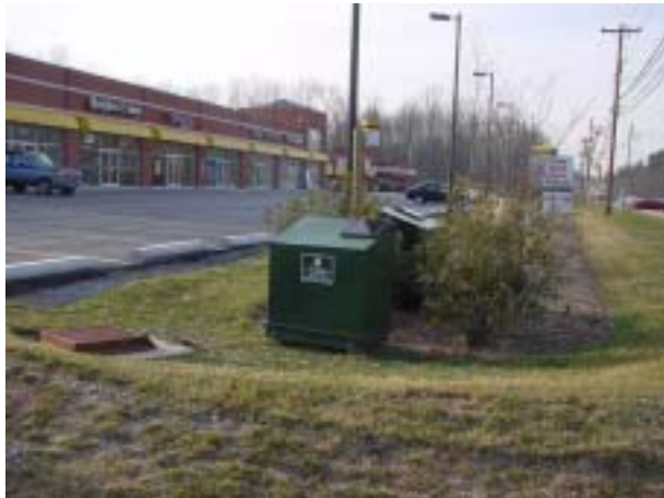
Figure 4. Bio-retention Cell #1 completed and outfitted for monitoring at Battleground Crossing Shopping Center in Greensboro, NC.
