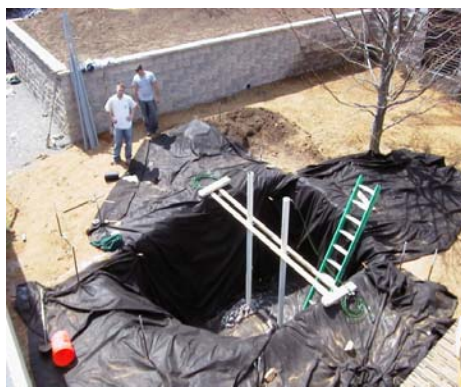
VU Infiltration Trench, (left) completion of trench excavation with geotextile fabric lining (note locations of the two monitoring wells) (right) completed infiltration trench (2005)
